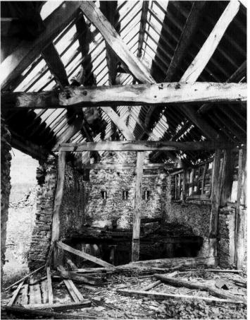
walled except on the east side where there is half-height timber framing; the twotiered square panels have an unusual form of infill or 'noggin' with horizontal planks slotted into grooves in the studs.
